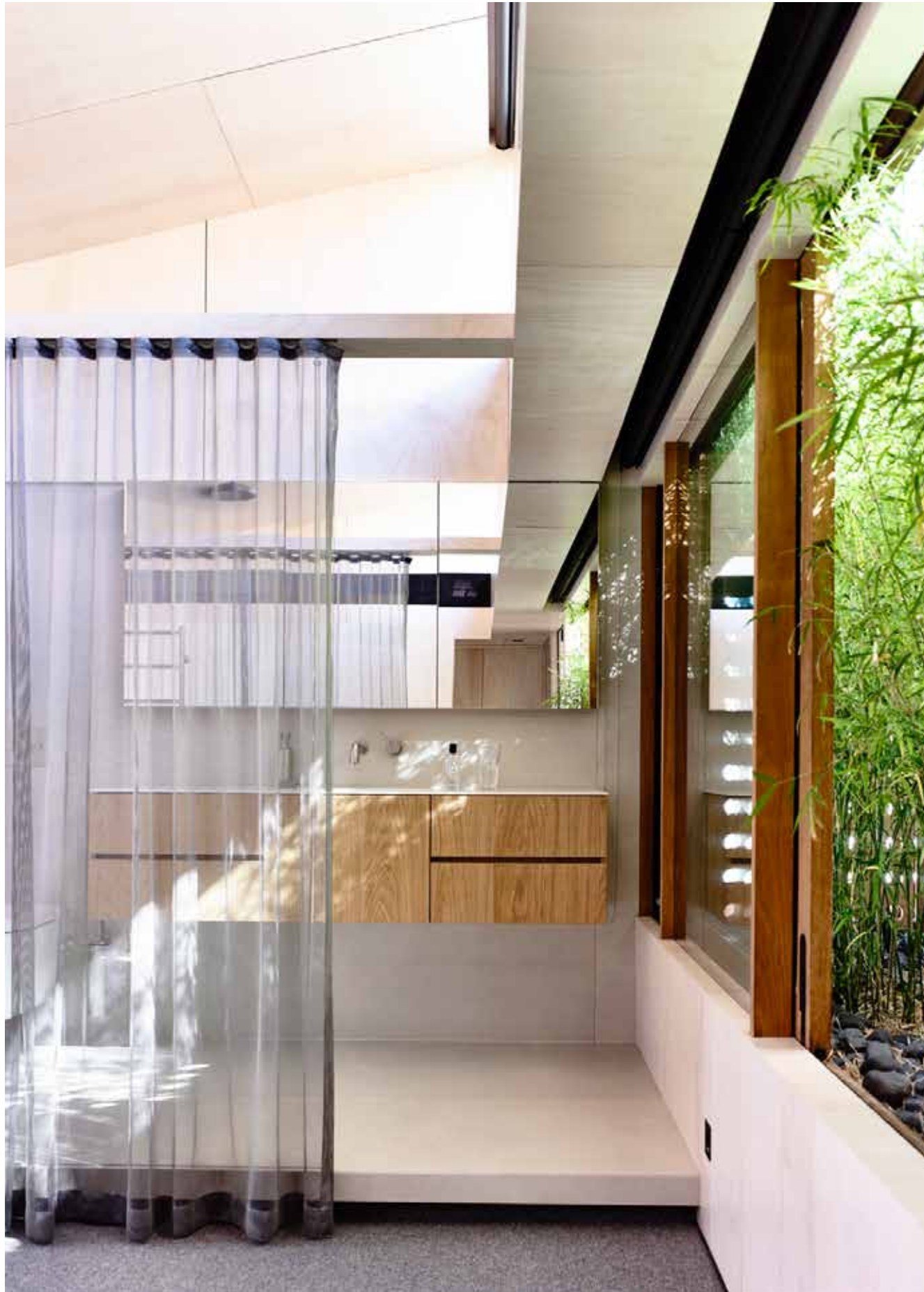
Above: Each ensuite has a mesh curtain but is otherwise open to the bedroom and raised garden to maximise the sense of space. Sloping ceilings allow space for high-level windows and maximum light penetration. Porcelain tiles line the bathroom floors and walls, the benchtop and sink are made of Corian, and joinery fronts are in rough-sawn American oak. Limed hoop pine lines the rest of the room.
